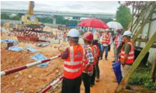
Site inspection with the certification body for ISO certification
