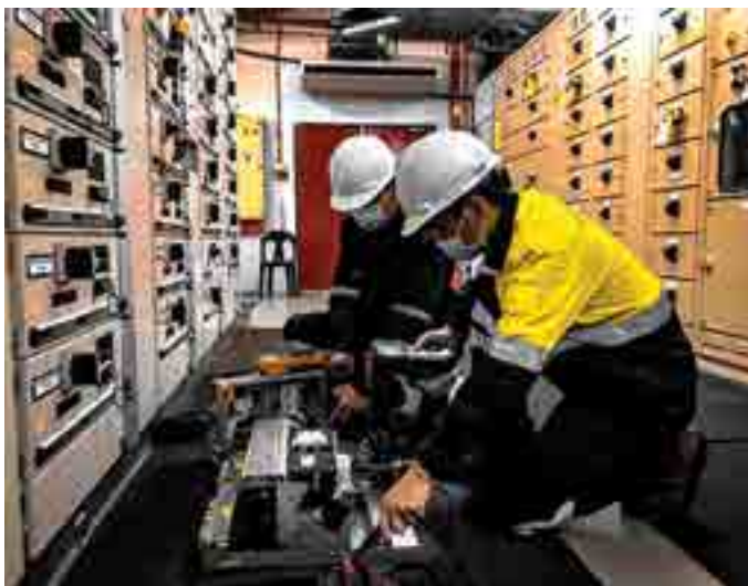
☞ Scheduled maintenance works on the gas turbine
