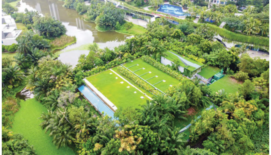
Forest City Sewage Treatment Plant, Johor Bahru, Johor that built underground is covered with landscape
