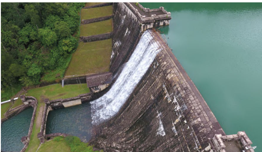
Gunong Pulai Reservoir is one of the main sources of the water supply system for part of residents in Johor Bahru and Pontian district, Johor state
