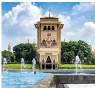
Clean and reliable water supply; contribute to health of communities and economy development
