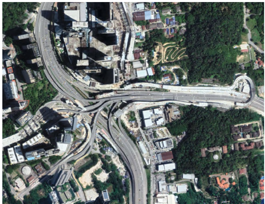
Damansara-Shah Alam Elevated Expressway (DASH) Penchala Interchange, one of Ranhill Bersekutu's remarkable highway projects
