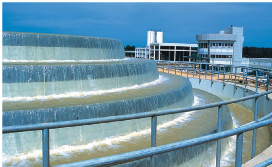
The aeration at Semangar Water Treatment Plant that is often used to eliminate carbon dioxide liberated by the treatment process
