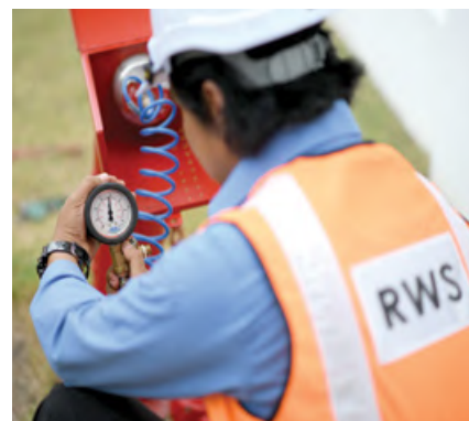
Ranhill Water Services technician at his best service; performing pressure monitoring
