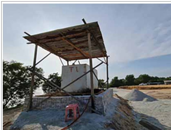
Proper basement for leakage control at diesel storage at E'Island Lake Haven
