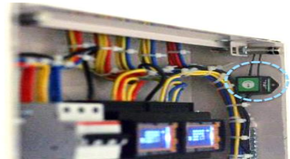
Installed sensors to track energy readings
