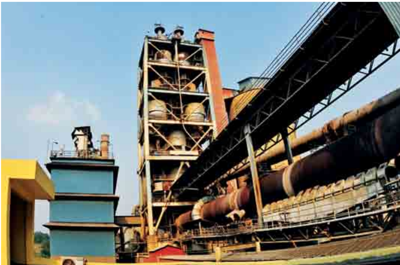
CMS Clinker's pre-heater and kiln.
