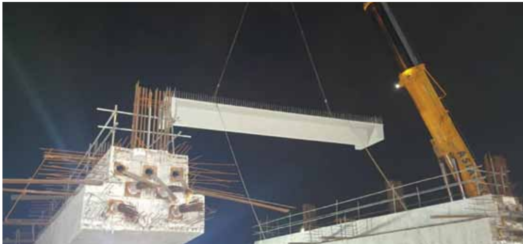
Picture: Precast Tee Slabs were supplied to Light Rail Transit Line 3 (LRT 3) from Bandar Utama to Johan Setia Package Eastern Corridor G305-Station 12 (Dato Menteri Station) and Station 14 (UiTM Shah Alam).
