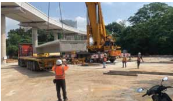
Picture: Precast RC T slab beams were supplied to customer namely Apex Communication Sdn Bhd for project LRT 3 Package GS05 Station 12 Dato Menteri Station and Station 14 UITM Shah Alam. The beams serve as slabs for LRT station.
