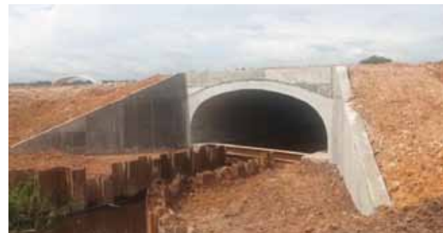
Picture: Precast Ribbed Arch Culverts RAC 6025 were supplied to customer namely IJM Construction for project West Coast Expressway Section 02. These culverts serve as a bridge for river crossing.
