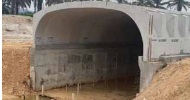
Picture: Precast Ribbed Arch Culverts RAC 12035 were supplied to customer namely Pembinaan Tetap Teguh for Kota Elmina Township as a bridge for river crossing.
