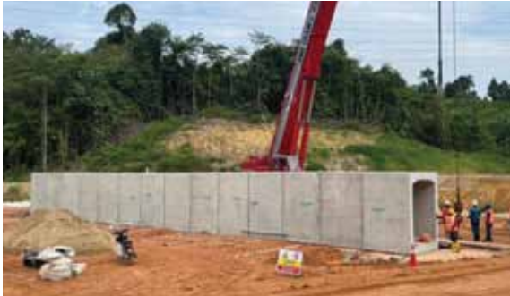
Picture: Precast Uni-Culverts were supplied to East Coast Rail Link ("ECRL") Section 5 to storm water drainage underneath ECRL railway.
