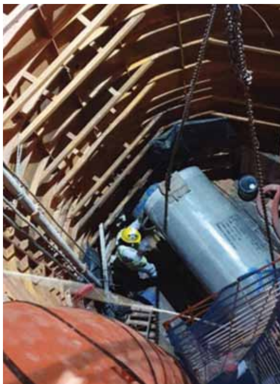
Picture: Mipipes® Polymer Concrete Jacking Pipe being lowered down the shaft in preparation for jacking at a Singapore site.
