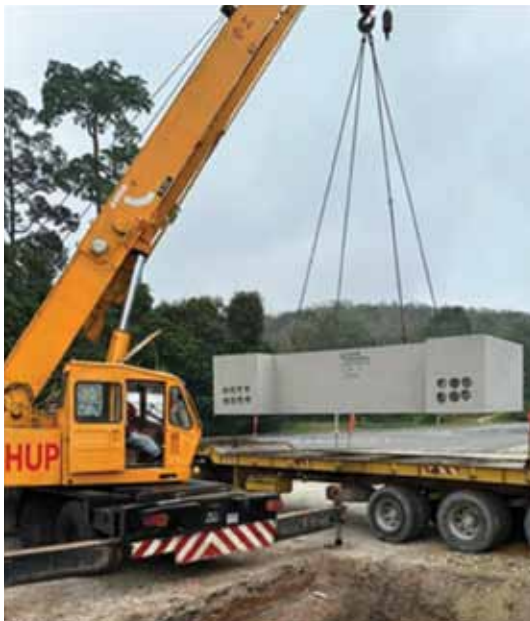
Picture: Installation of Precast Tenaga Nasional Berhad (“TNB”) Compact Substation Plinth at site
