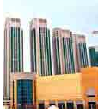
The Central Waste Handling Facility at Marina Square, Al Reem Island, Abu Dhabi
