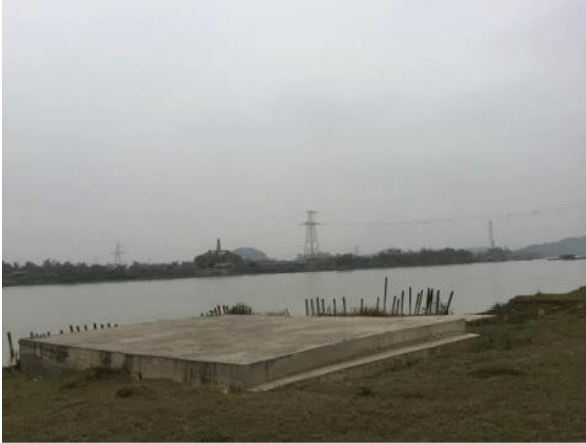
Fig 1: The coal jetty site (March'16)
