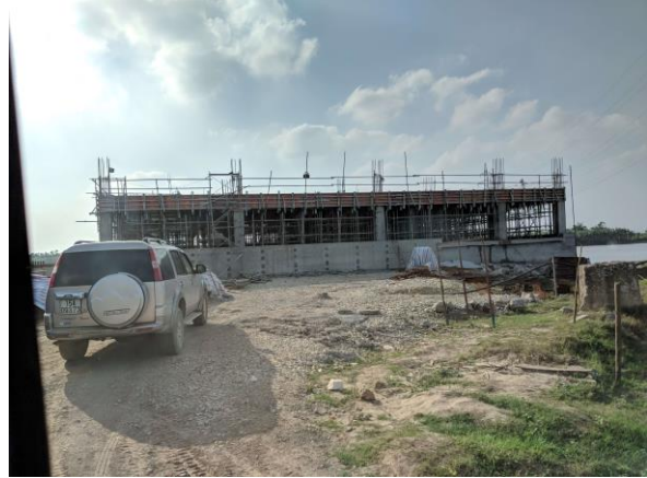
Fig 2: The coal jetty site - 1 (Jan'18)
